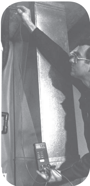
FIGURE 48 TEMPERATURE RISE MEASUREMENT
