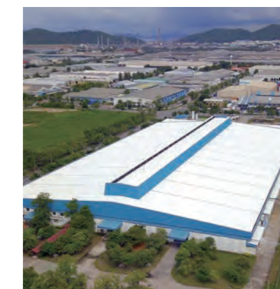
Fujitsu General (Thailand) Co., Ltd. (Thailand) Factory-2
