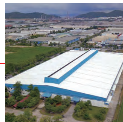
Fujitsu General (Thailand) Co., Ltd. (Thailand) Factory-2
