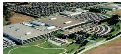
North America R&D Center (USA)
