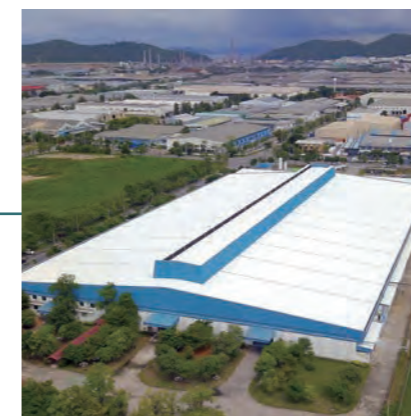
Fujitsu General (Thailand) Co., Ltd. (Thailand) Factory-2
