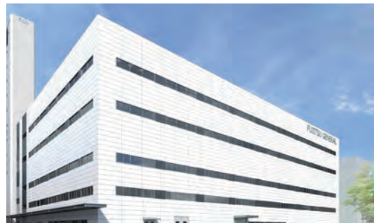
Technology research building (Japan)
