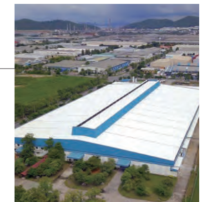
Fujitsu General (Thailand) Co., Ltd. (Thailand) Factory-2
