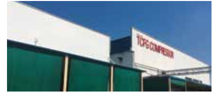
TCFG Compressor (Thailand) Co., Ltd. (Thailand)
