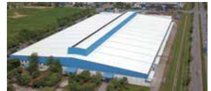
Fujitsu General (Thailand) Co., Ltd. (Thailand) FACTORY-2
