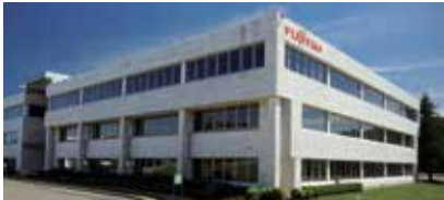
North America Corporate HQ and Training Center Fujitsu General America (Pine Brook, NJ, USA)
