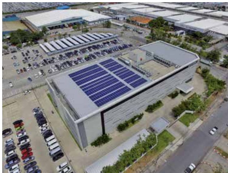
Solar panels newly installed on the rooftop of Fujitsu General Air Conditioning R&D (Thailand) Co.,Ltd.
