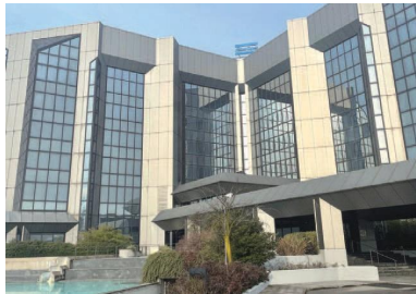
(Left) Building where FG (ITALIA) resides
