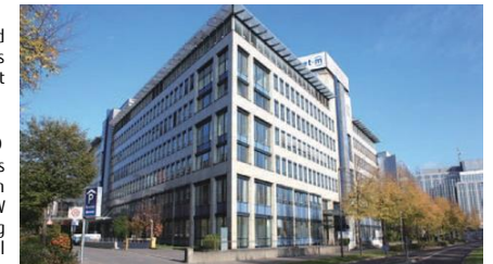
Building where FG(EURO) resides
