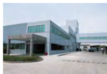
FUJITSU GENERAL (SHANGHAI) CO., LTD. Technical Center
