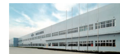
Fujitsu General Central Air-conditioner (Wuxi) Co., Ltd. (China)
