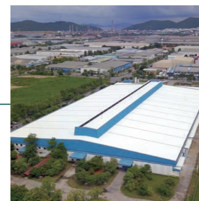
Fujitsu General (Thailand) Co., Ltd. (Thailand) Factory-2
