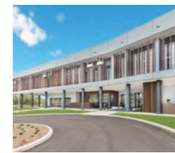
Fujitsu General (Aust.) Pty Ltd. (Australia)
